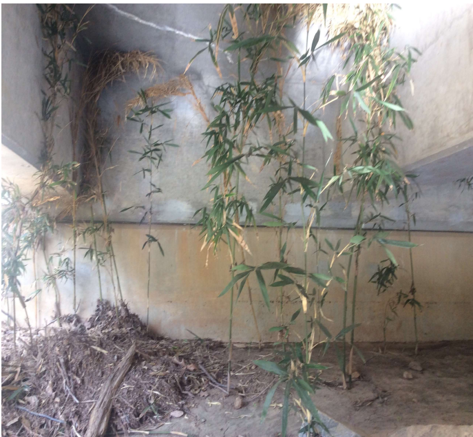
PHOTO 1 Description Bent 6 west end of bridge canes growing under bridge.
